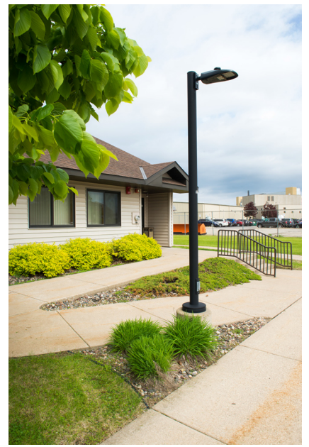
Swift Creek apartments 20190522 03.jpg
